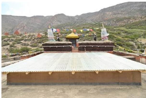
Figure 4: The roofing of the courtyard largely completed.
