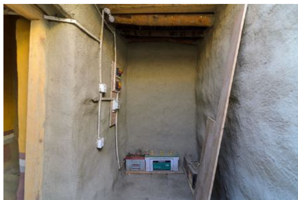
Figure 21: Battery storage and main electrical power control in the room that also allows access to the roof.
