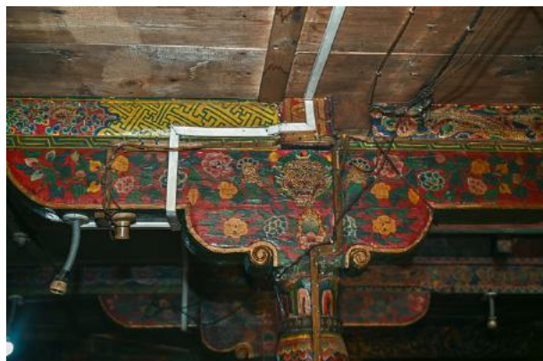
Figure 17: An example of the multiple, partially dysfunctional lighting systems used previously in the assembly hall.
