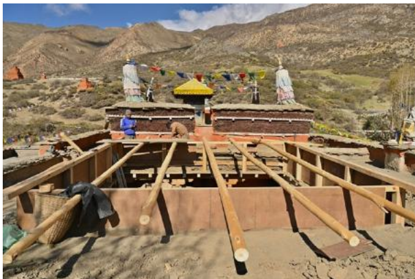
Figure 2: The construction of the frame for the roofing of the courtyard.
