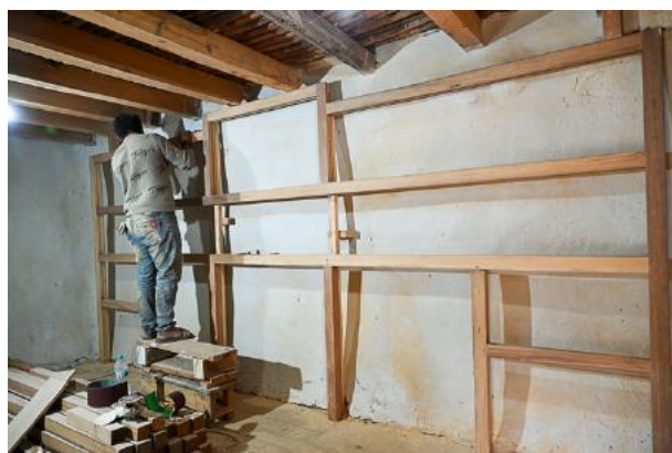
Figure 12: The frame for the Arhat panels under construction.
