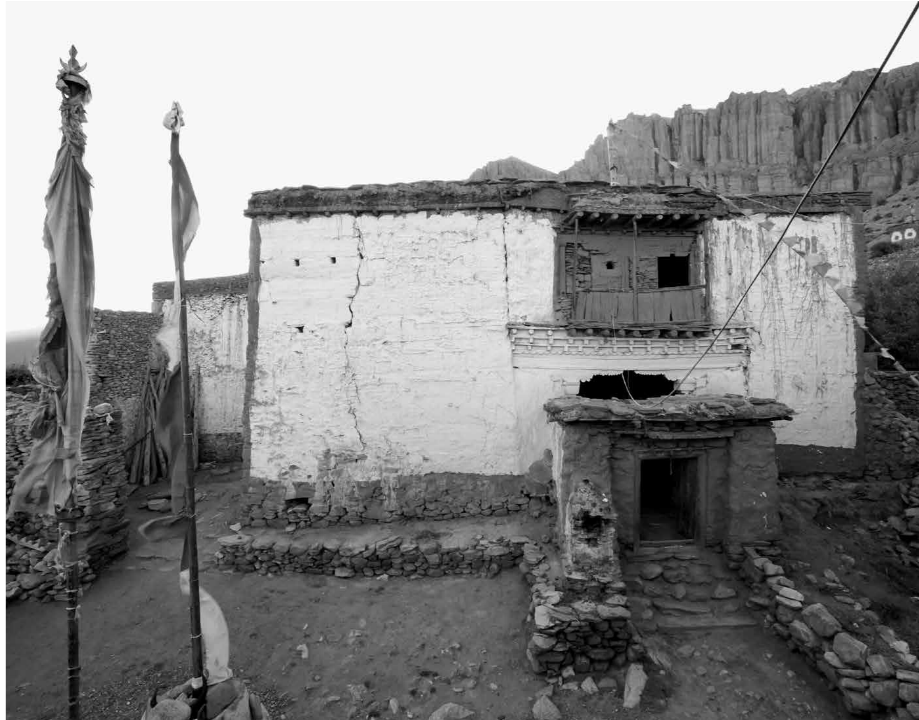
PRINCIPAL FACADE FACING EAST 2022
