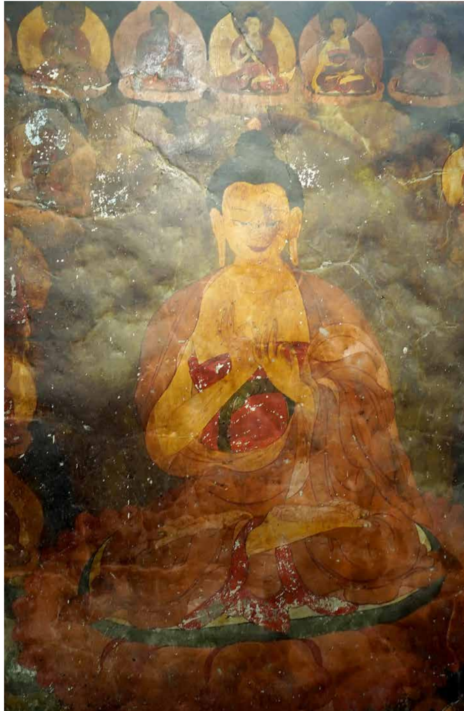
WALL PAINTING DEPICTING BUDDHA Flaking of the paint layer is an indication of damp walls.
