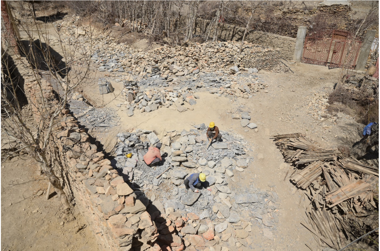
Figure 25: Preparation of the stone panels for the drainage.
