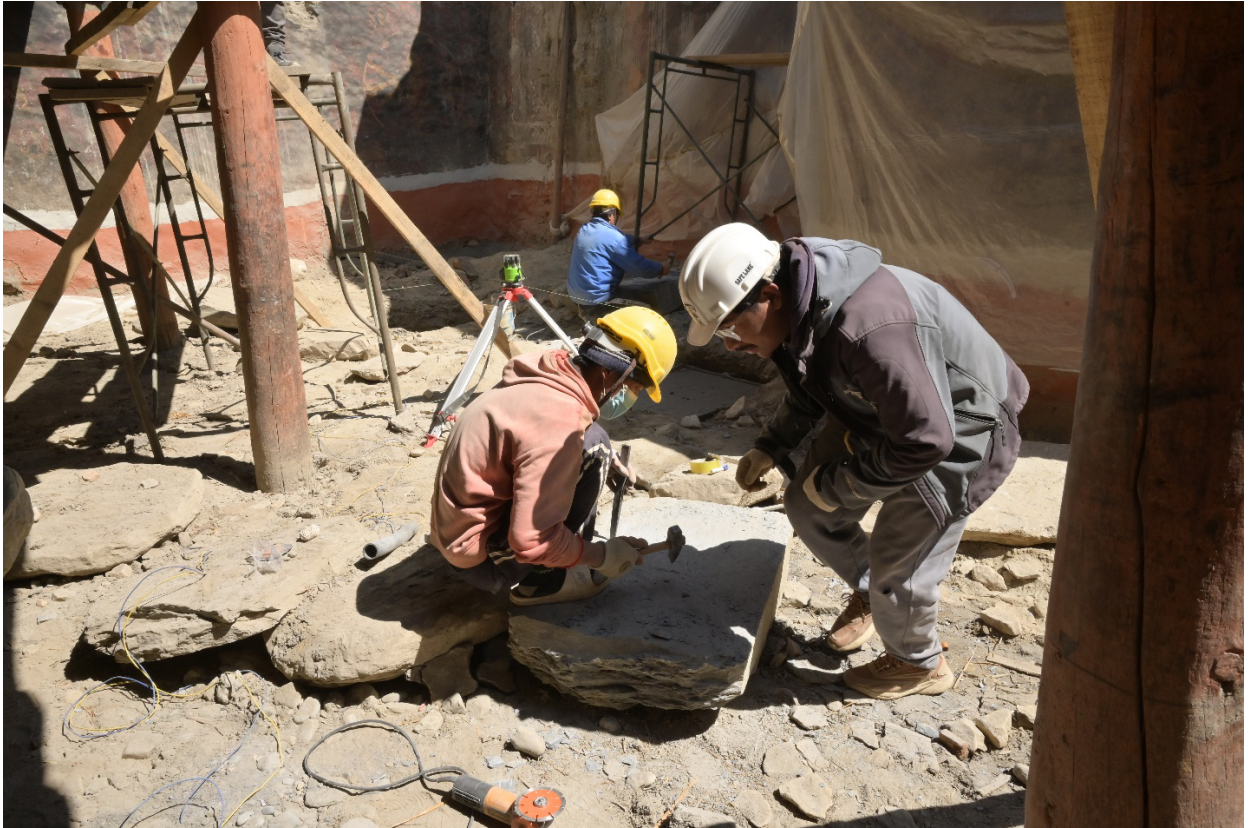
Figure 24: Preparation of a new stone base for one of the columns.
