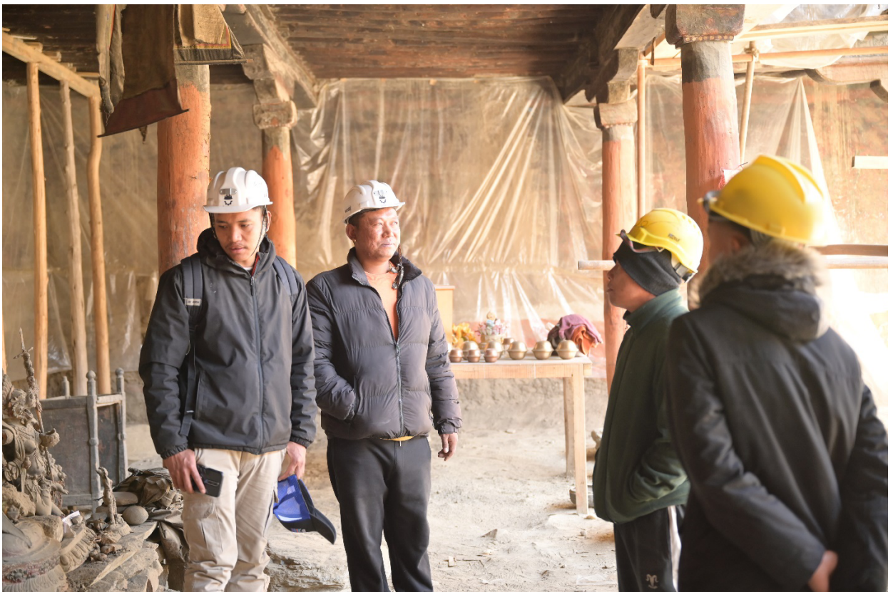
Figure 27: Inspection of the work on site.
