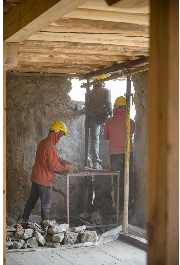
Figure 6: Supporting the cross beams of the northeast corner on the ground floor level.
