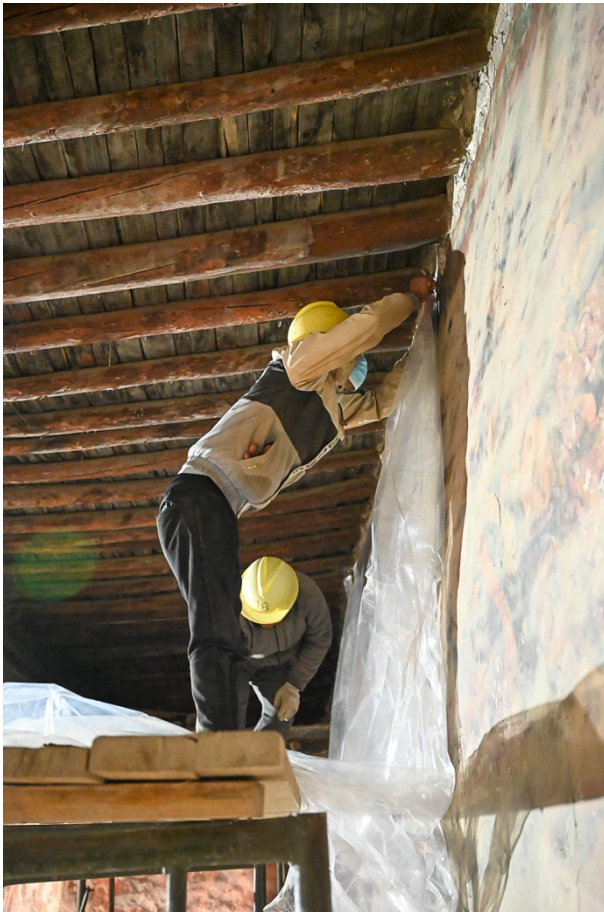
Figure 17: Attaching the plastic sheets.
