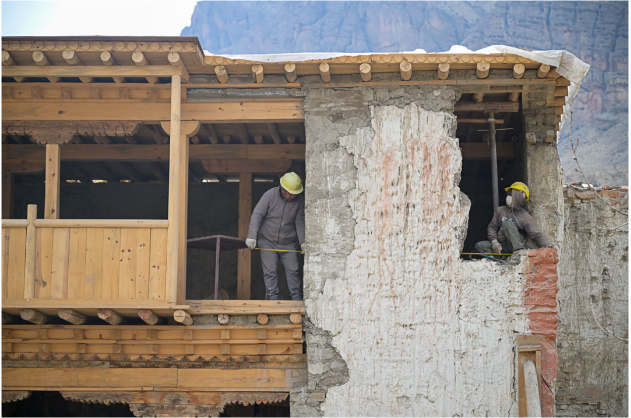
Figure 8: The upper part of the northeast corner after dismantling.
