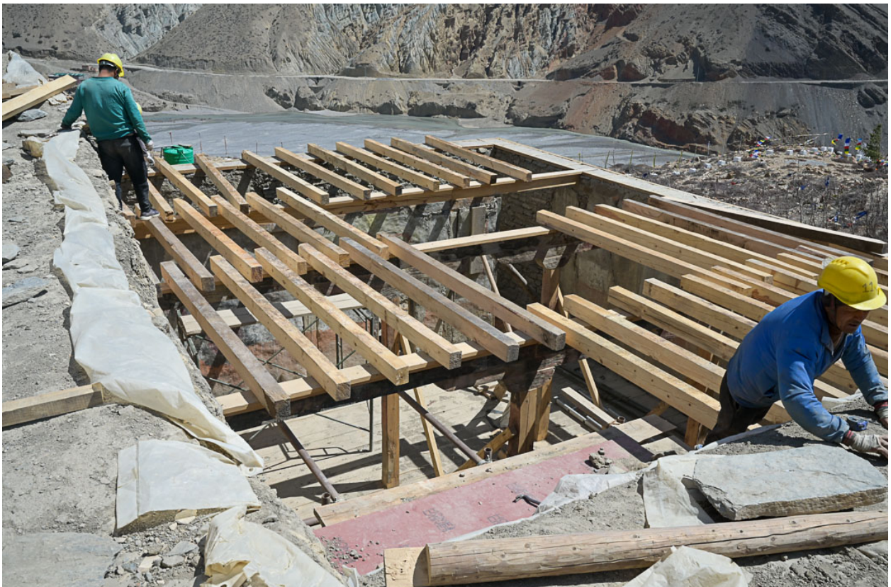
Figure 14: Placing the joists above the south wing.
