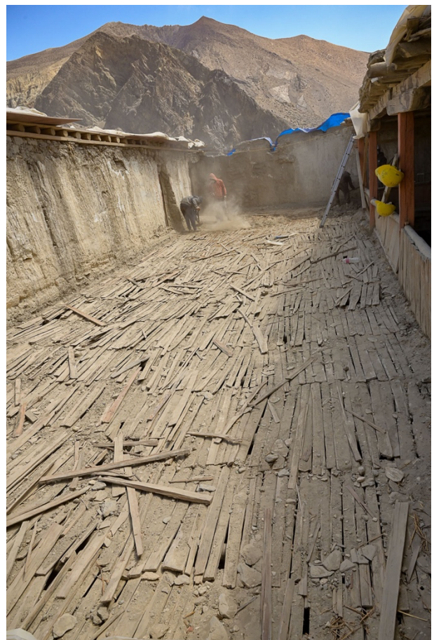
Figure 19: Removal of the roof above the Assembly Hall, including the plastic sheets added in an earlier village restoration.
