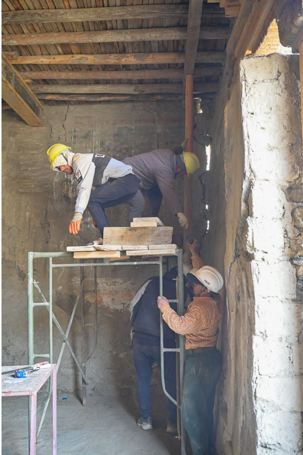
Figure 6: Supporting the cross beams of the northeast corner on the ground floor level.
