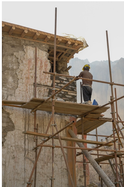
Figure 9: Placing the lowest wall tie on the upper floor of the northeast corner.
