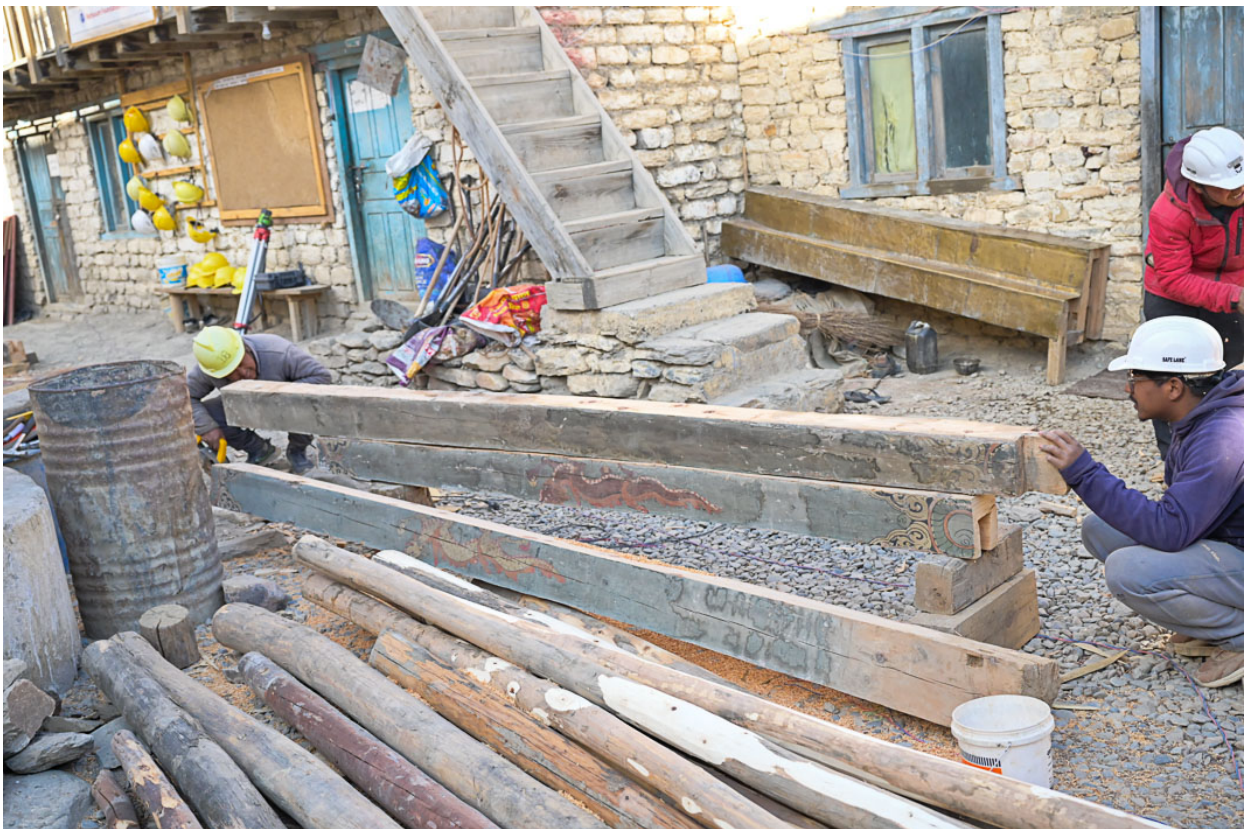
Figure 23: Inspection of the original wooden beams to prepare them for reuse.
