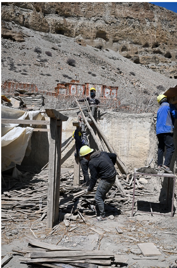
Figure 20: Dismantling the support structure on the upper level.
