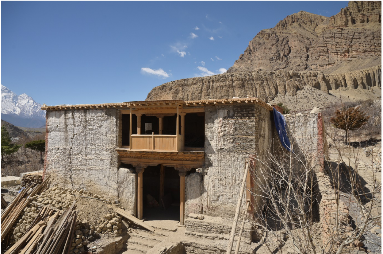
Figure 1: Photo taken on March after renovation of corner wall.
