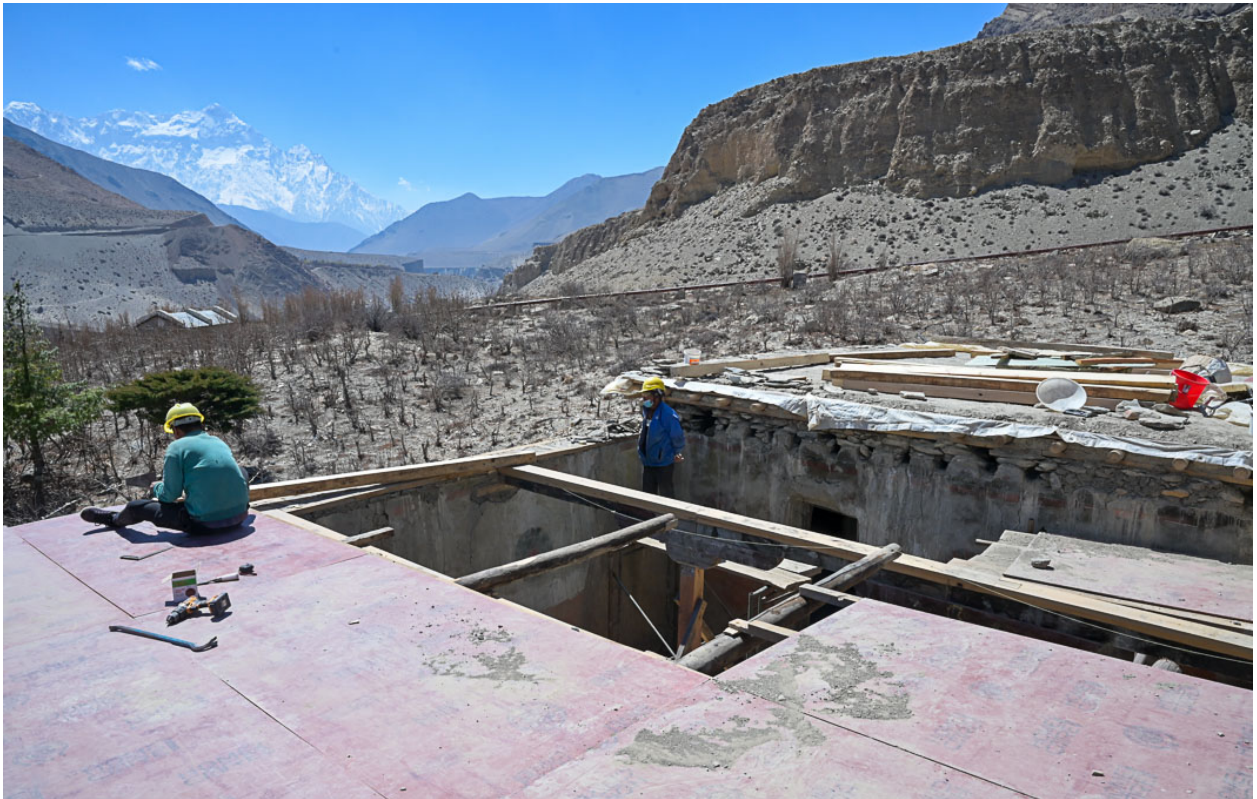
Figure 13: Removing the temporary roof of the south wing.
