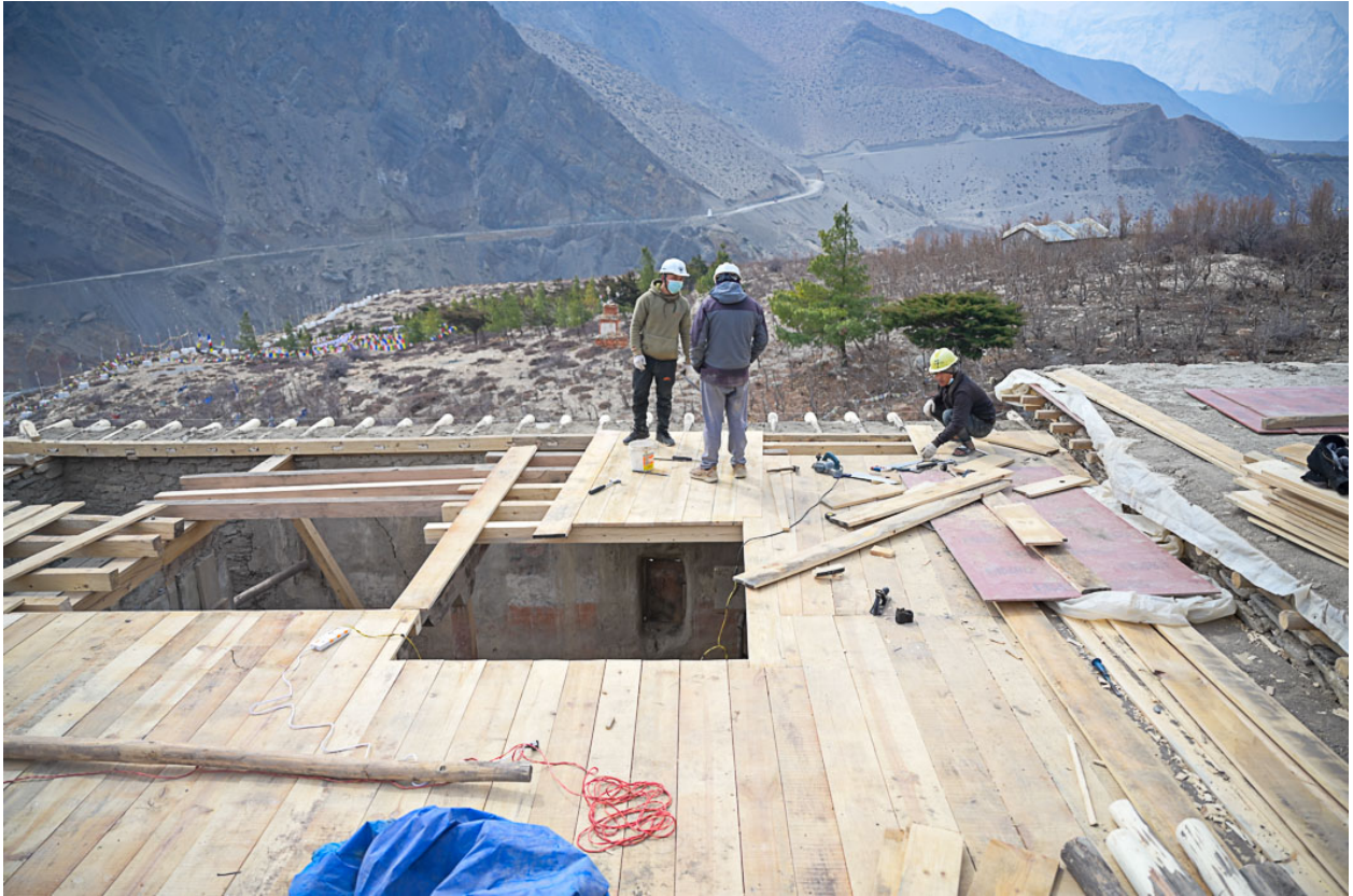
Figure 15: Adding the planking to the roof of the south wing.
