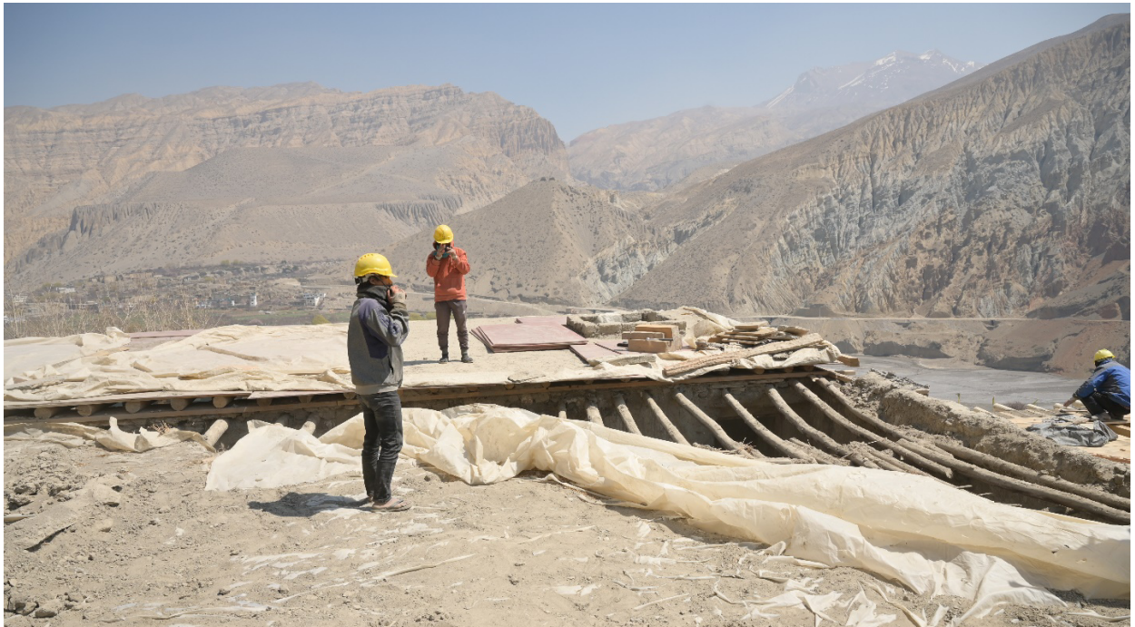
Figure 19: Removal of the roof above the Assembly Hall, including the plastic sheets added in an earlier village restoration.
