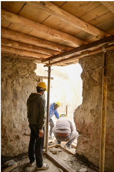
Figure 9: Placing the lowest wall tie on the upper floor of the northeast corner.
