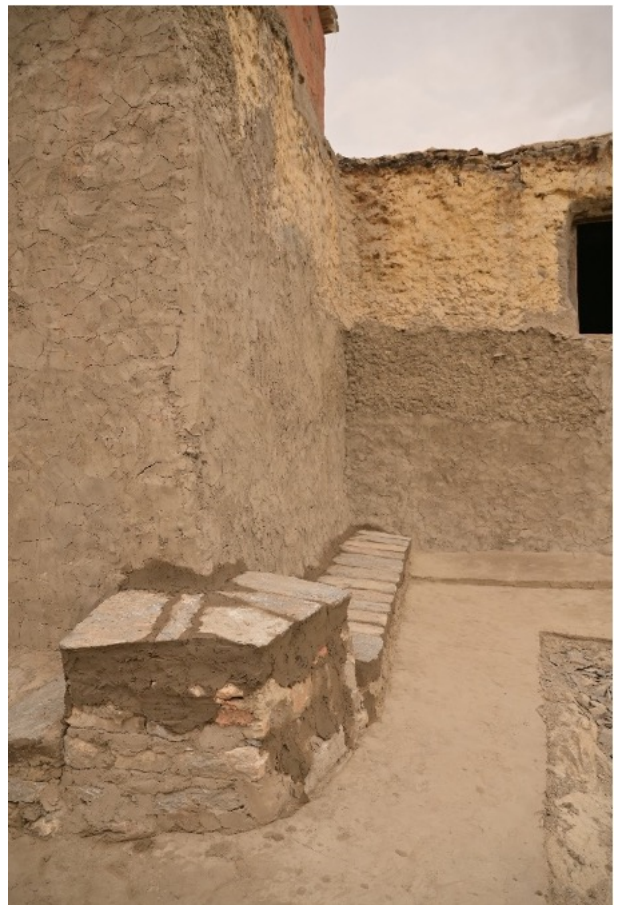
Figure 52: The mud layered between newly constructed stonewall and the drainage maintaining a slope.
