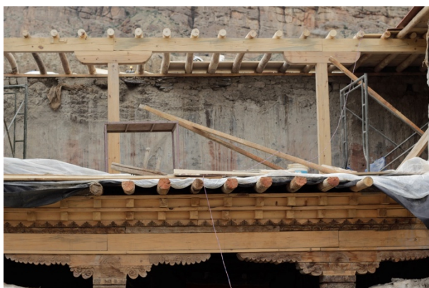
Figure 21: Zoom view of wooden structural members of the first floor.
