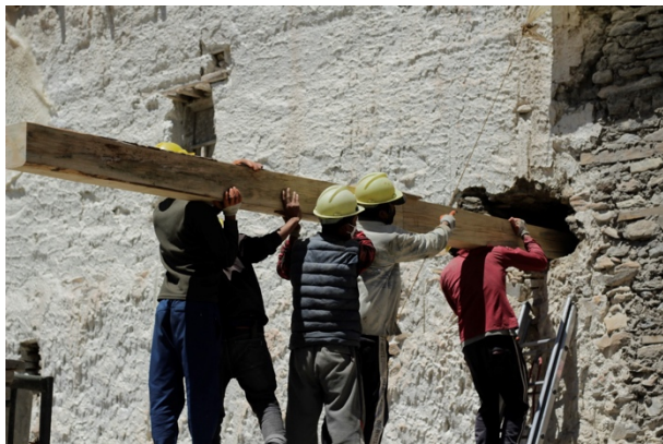
Figure 42: Inserting the new beam to replace old one through a hole in the wall.
