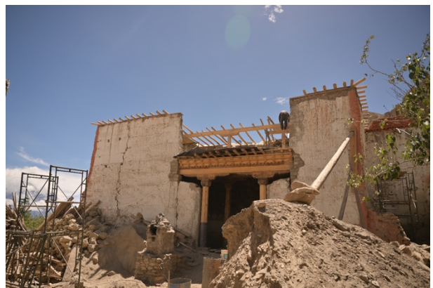
Figure 18: Assembling the central wooden structure at the level above the Entry Hall.
