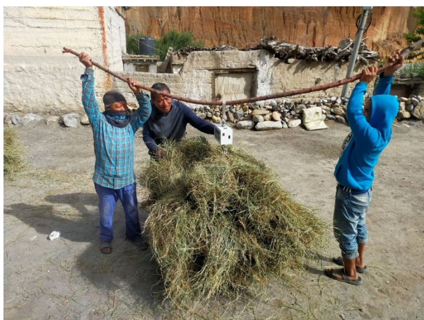
Figure 2: Weighing a bundle of dry grass purchased from the villagers to mix with mud for the adobe bricks.
