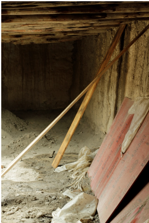
Figure 69: Plastic sheets and plywood used to prevent water affecting the wall paintings on the floor underneath.
