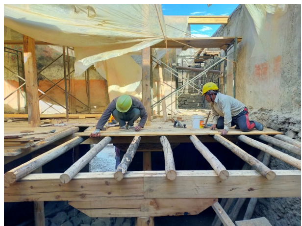
Figure 43: The ground floor level with half of the wooden structure already replaced.
