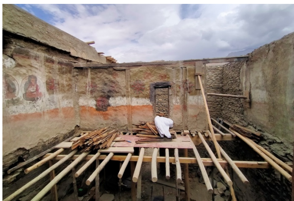
Figure 44: Gradually progressing from the ground floor to the first floor.
