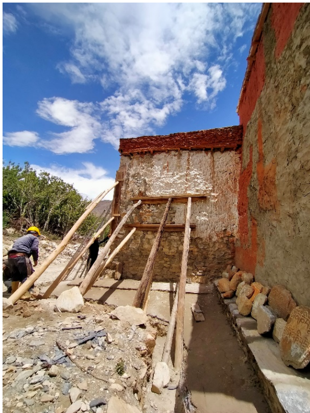
Figure 58: First the wall was shored up to prepare the dismantling from the top.
