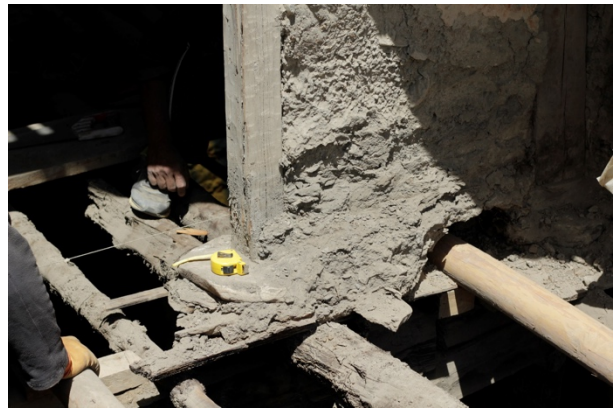
Figure 37: Adding additional support posts to hold up the walls on the upper floor.
