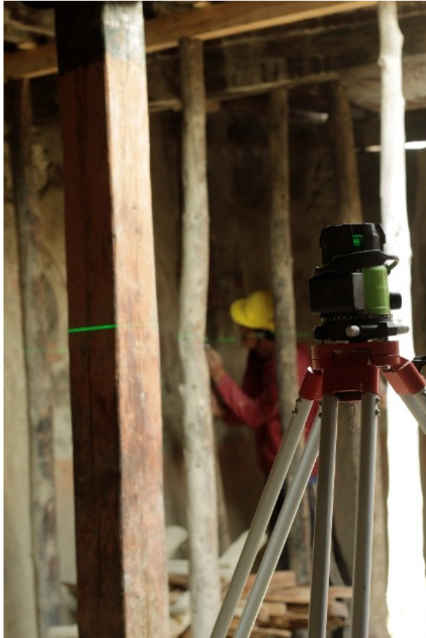
Figure 36: Taking the levels with laser before dismantling the wooden structure.
