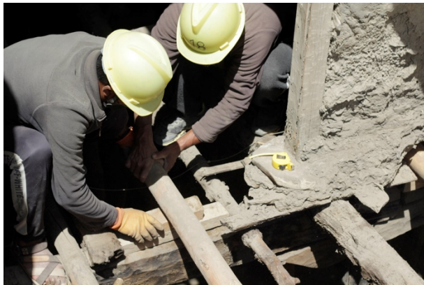
Figure 38: Replacing the old joist with new one maintaining the level.
