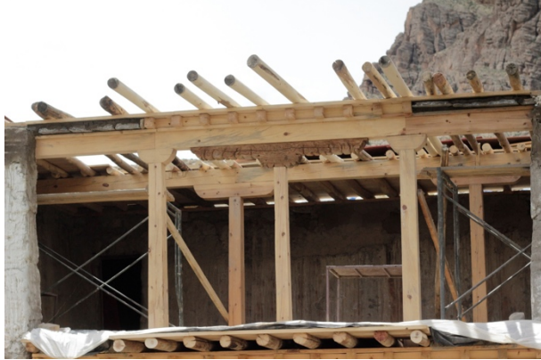
Figure 23: Placing the joist between the central beam and the porch area.
