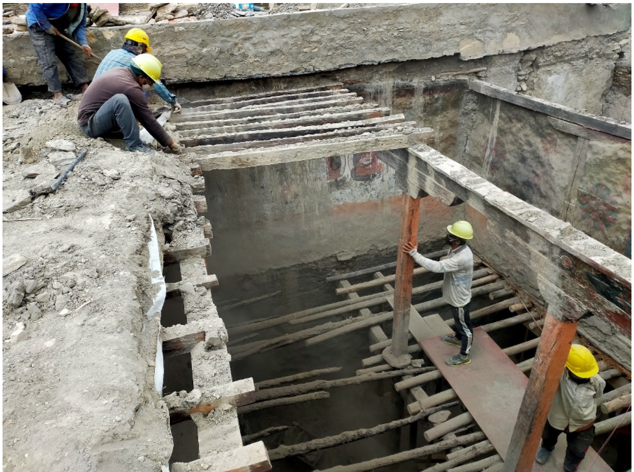
Figure 35: Dismantling the roof above the painted room in progress.
