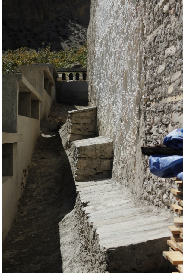
Figure 54: Section of the foundation wall on the south side after finishing the layer of mud and stone slate.
