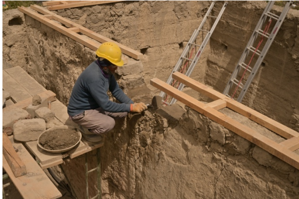
Figure 17: Leveling for the wooden plate to place the central beam.
