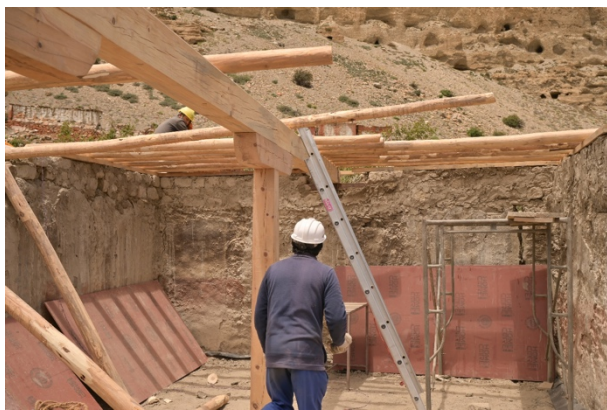
Figure 19: Placing the joist according to their shape and sizes.
