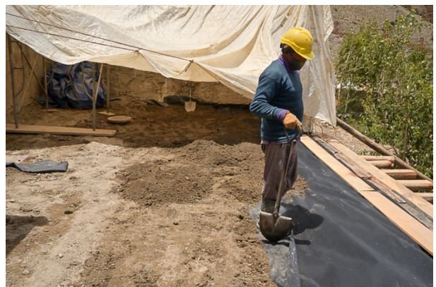
Figure 13: Adding a mud layer on top of a special fabric to build the floor of the upper storey.
