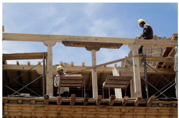
Figure 20: View from the front while placing the joists on the level above the Entry Hall.
