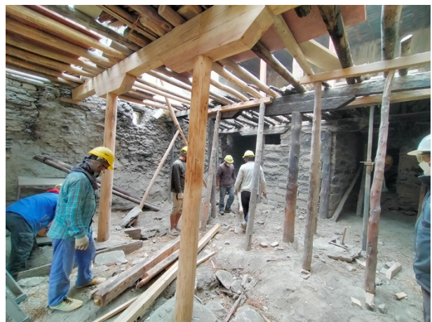
Figure 42: Inserting the new beam to replace old one through a hole in the wall.
