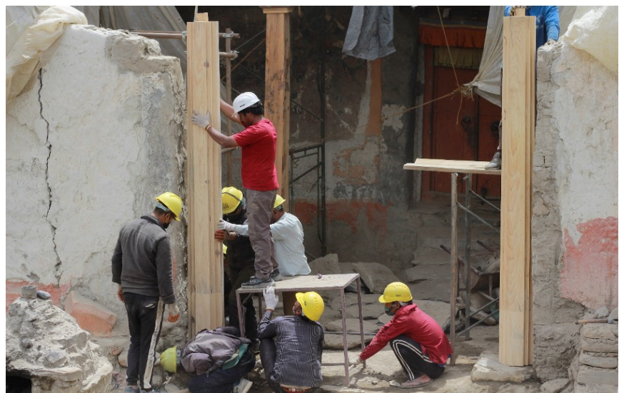
Figure 5: Placing the front column on the bed stone with a projection connecting it to it.
