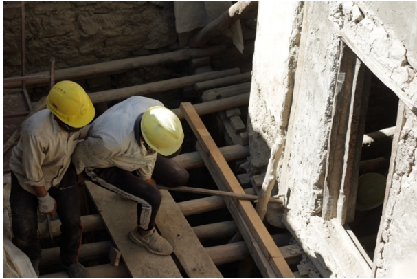
Figure 40: Placing the joist under the first floor column and partition wall.
