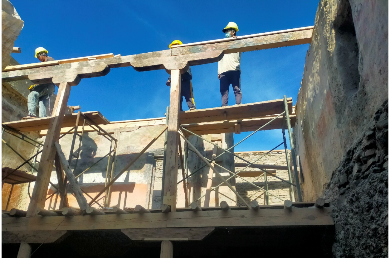
Figure 46: Reassembling the old wooden structure after repair.
