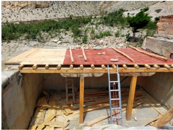
Figure 28: The structural wooden members for the roofing of the southwestern room prepared for assemblage.
