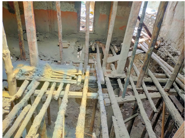
Figure 32: Laying the wooden ties to tie to connect the old and new stone walls.
