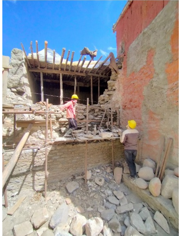
Figure 63: Construction of the new wall along the lower section of the wall and connecting it with the old one.
