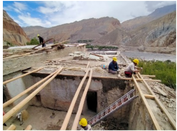
Figure 28: The structural wooden members for the roofing of the southwestern room prepared for assemblage.
