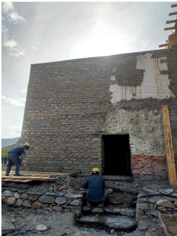
Figure 47: Constructing the stair to access the ground floor of southern part of Gönpa.
