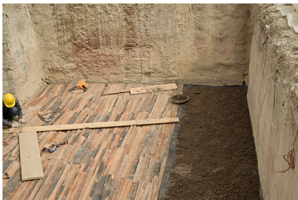
Figure 13: Adding a mud layer on top of a special fabric to build the floor of the upper storey.
