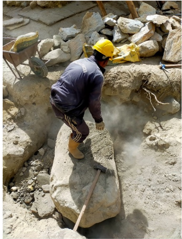
Figure 54: Section of the foundation wall on the south side after finishing the layer of mud and stone slate.
