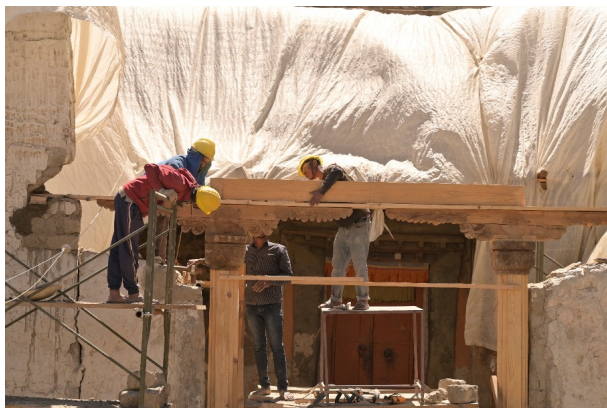
Figure 9: Arranging the positioning of the central beam as per measurements.
