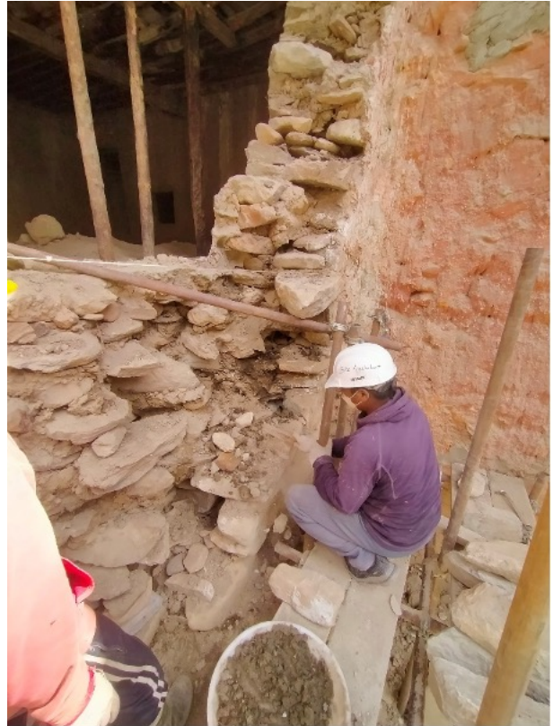
Figure 60: An extra wall was constructed in front of the problematic wall as support.
