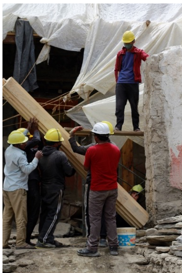
Figure 5: Placing the front column on the bed stone with a projection connecting it to it.
