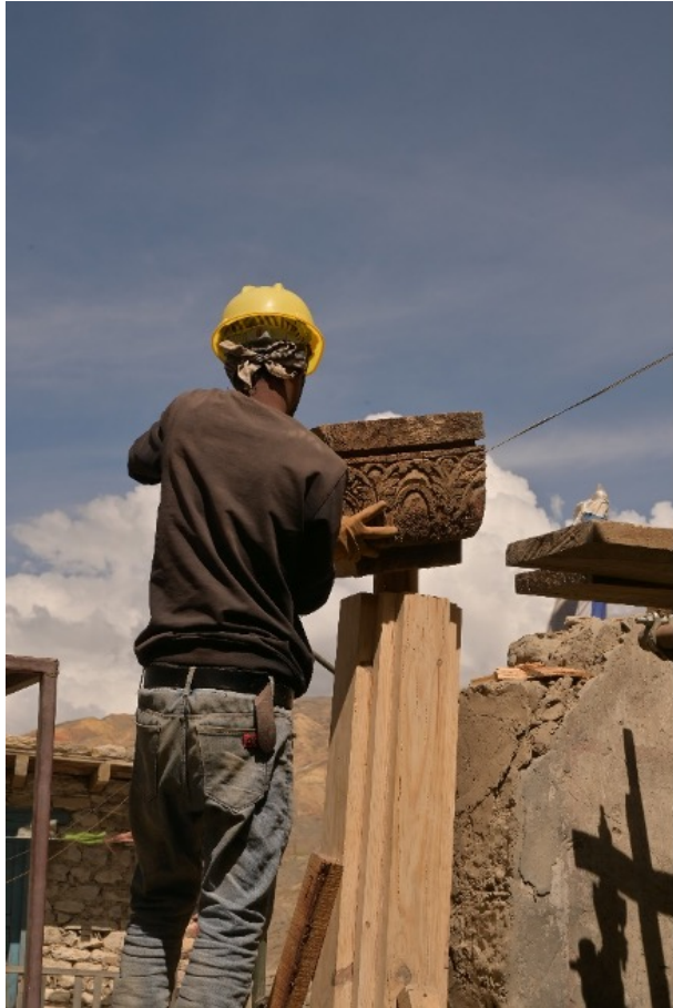
Figure 7: Connecting the old capital base to the new column.
