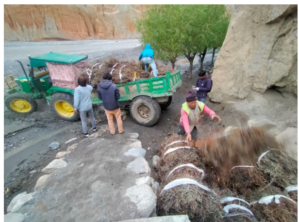
Figure 2: Weighing a bundle of dry grass purchased from the villagers to mix with mud for the adobe bricks.
