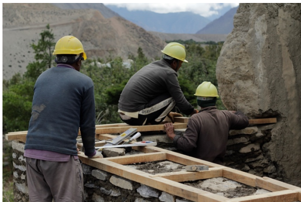
Figure 32: Laying the wooden ties to tie to connect the old and new stone walls.
