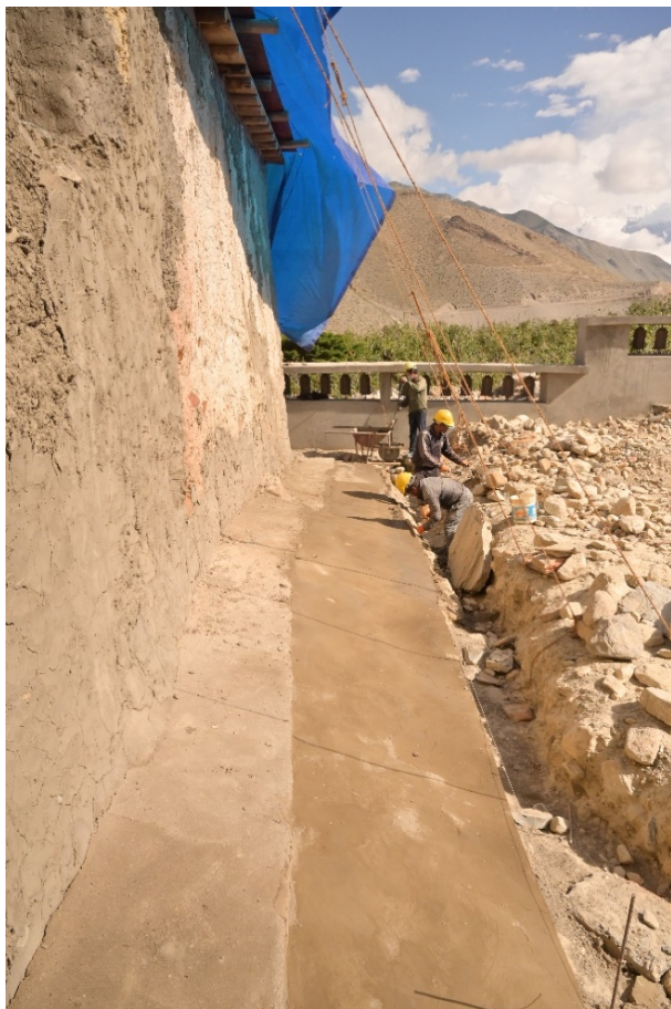
Figure 52: The mud layered between newly constructed stonewall and the drainage maintaining a slope.
