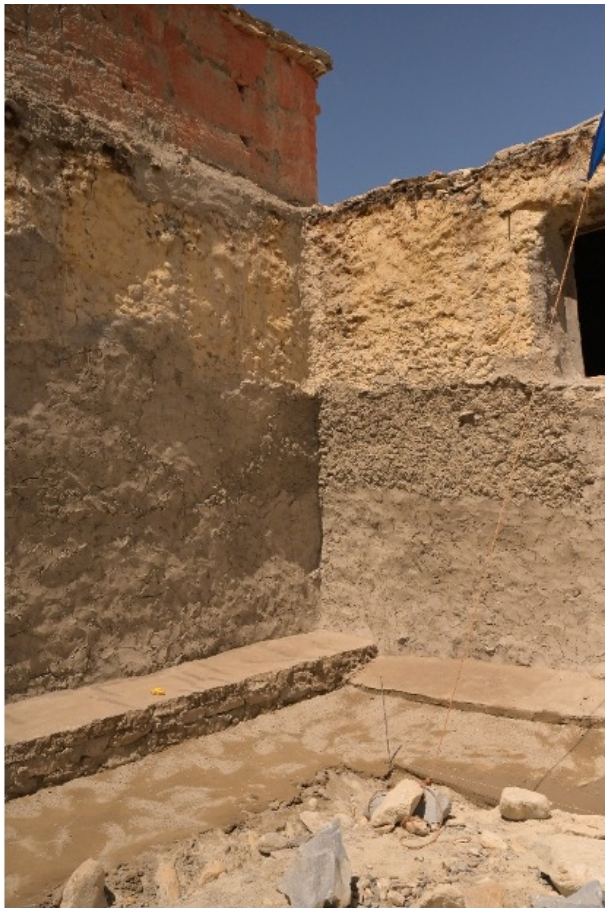
Figure 49: Covering the foundation support wall and the ground in front of it with mud.
