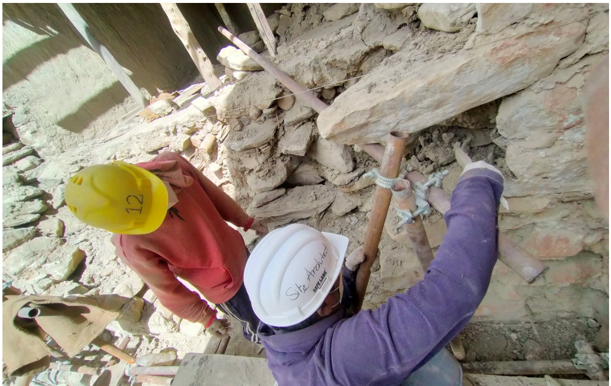
Figure 62: Supporting a large stone from the original wall that can serve as connector between the old and new walls.
