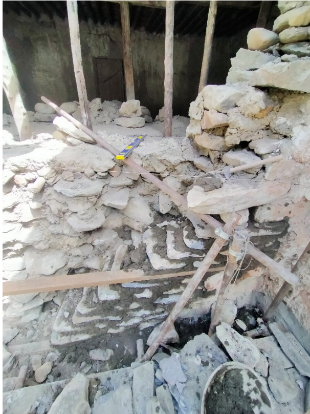
Figure 63: Construction of the new wall along the lower section of the wall and connecting it with the old one.
