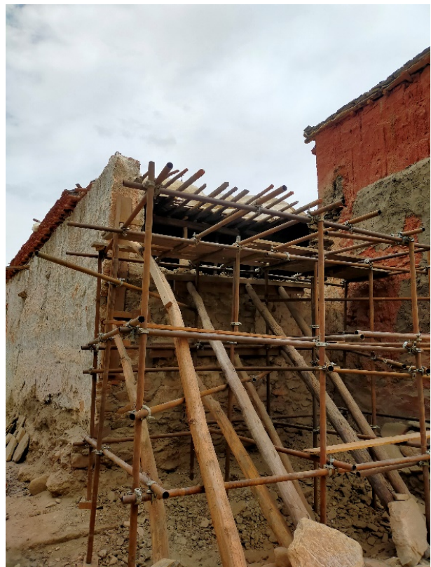
Figure 58: First the wall was shored up to prepare the dismantling from the top.
