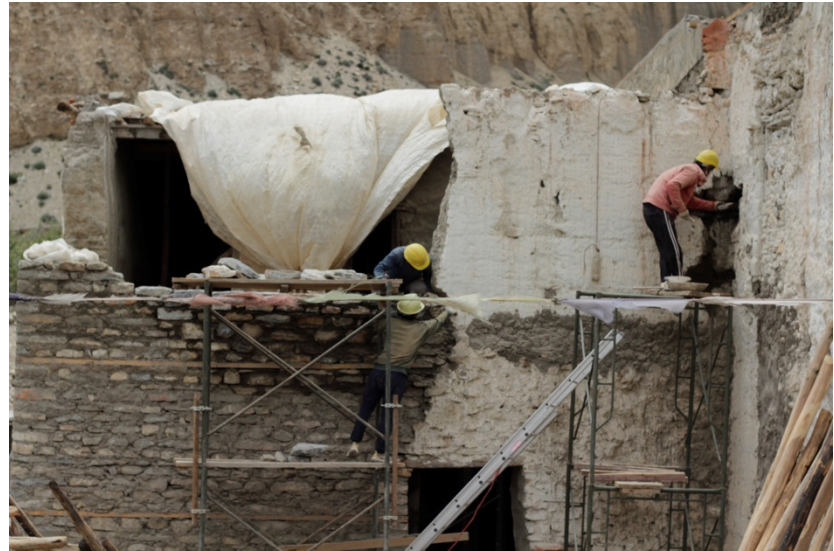
Figure 30: Repairing the old wall in front of the southern building with wooden ties.
