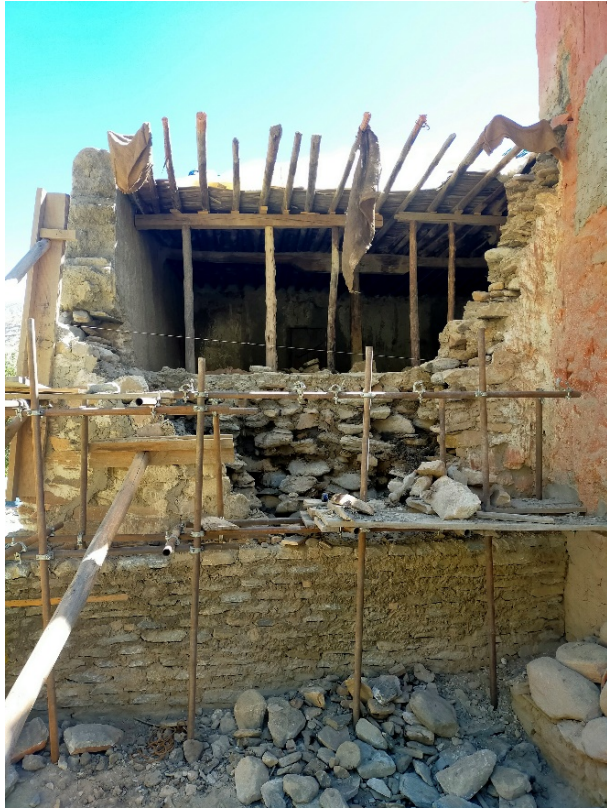
Figure 60: An extra wall was constructed in front of the problematic wall as support.
