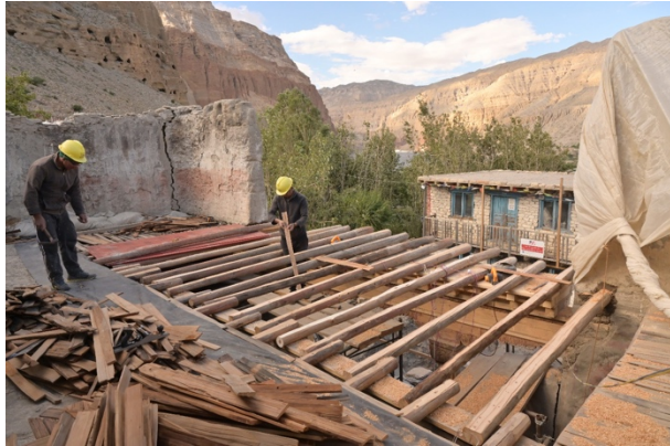
Figure 11: Arranging the old joist at Entry Hall with given measurement.
