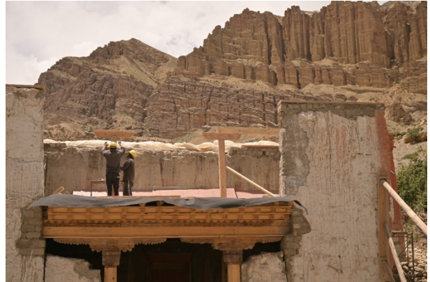
Figure 18: Assembling the central wooden structure at the level above the Entry Hall.
