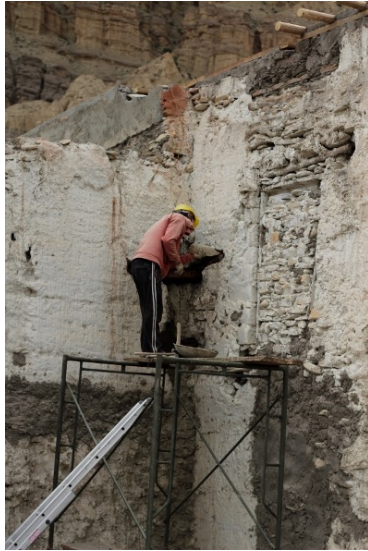
Figure 30: Repairing the old wall in front of the southern building with wooden ties.
