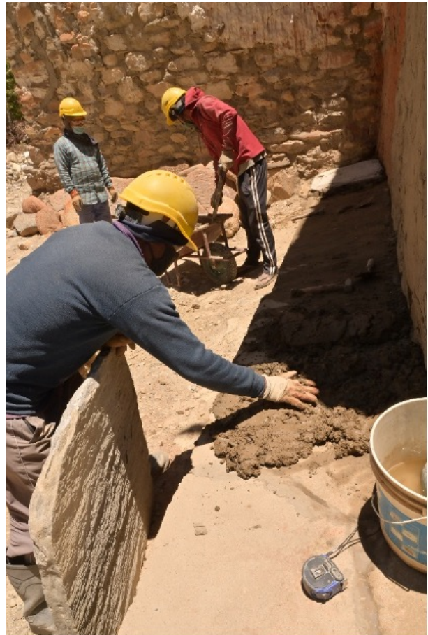
Figure 49: Covering the foundation support wall and the ground in front of it with mud.
