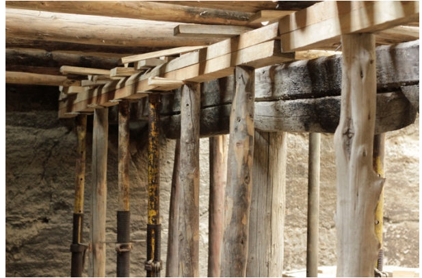
Figure 41: Supports installed to preserve the painted partition wall above during reconstruction.
