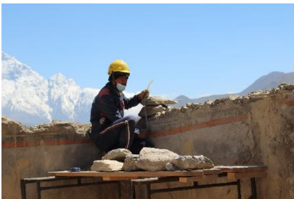
Figure 34: Leveling the top of the wall to enable the installation of a wall tie for seismic strengthening.
