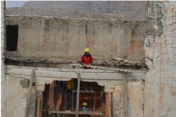
Figure 7: then the lower part of the porch was dismantled as well.
