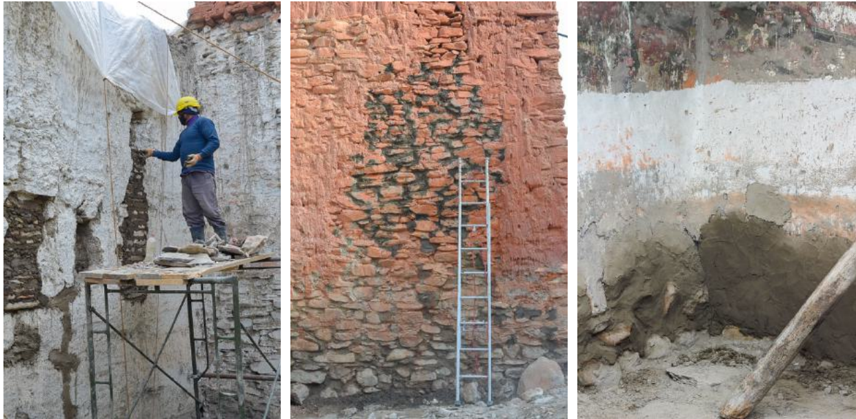
Figure 47: Repairing sections of the outer wall.
