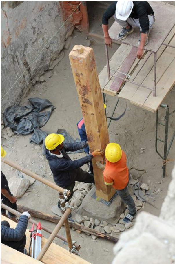
Figure 15: The old pillar with extension is placed on the new bedrock for reconstruction.
