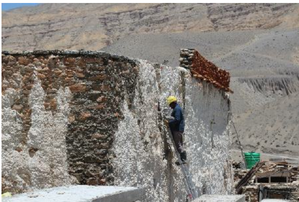
Figure 46: Repairing the areas of wall where the stones are revealed.
