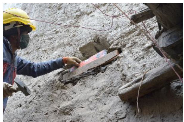
Figure 11: The original beam holding the porch was lengthened by adding a new bottom section.
