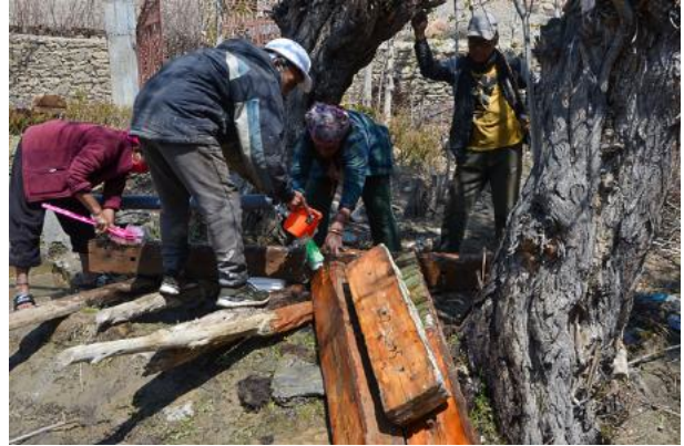
Figure 13: All original wooden members were cleaned and prepared for reconstruction, as demonstrated by Thomas Schrom here.
