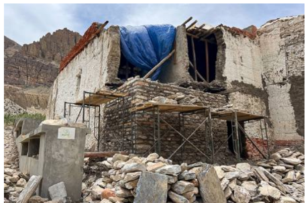
Figure 44: The construction of the wall close to reaching the ceiling of the ground floor.
