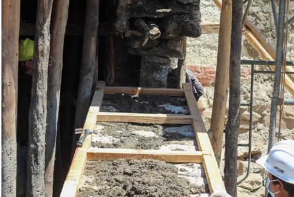
Figure 42: The wooden wall tie for seismic strengthening.
