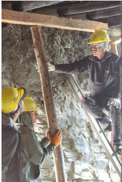
Figure 37: Adding supports in the interior before dismantling the south-eastern corner.
