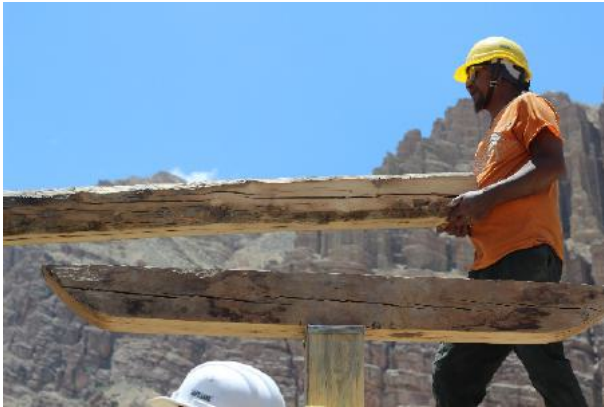
Figure 32: Assembling an old capital on top of a new beam on the top floor, note that their connection is reinforced.
