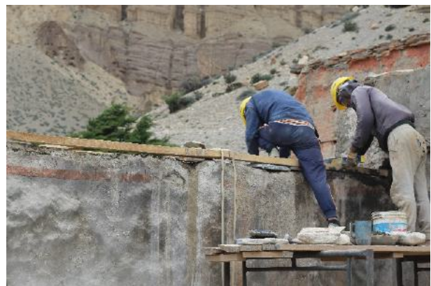
Figure 34: Leveling the top of the wall to enable the installation of a wall tie for seismic strengthening.
