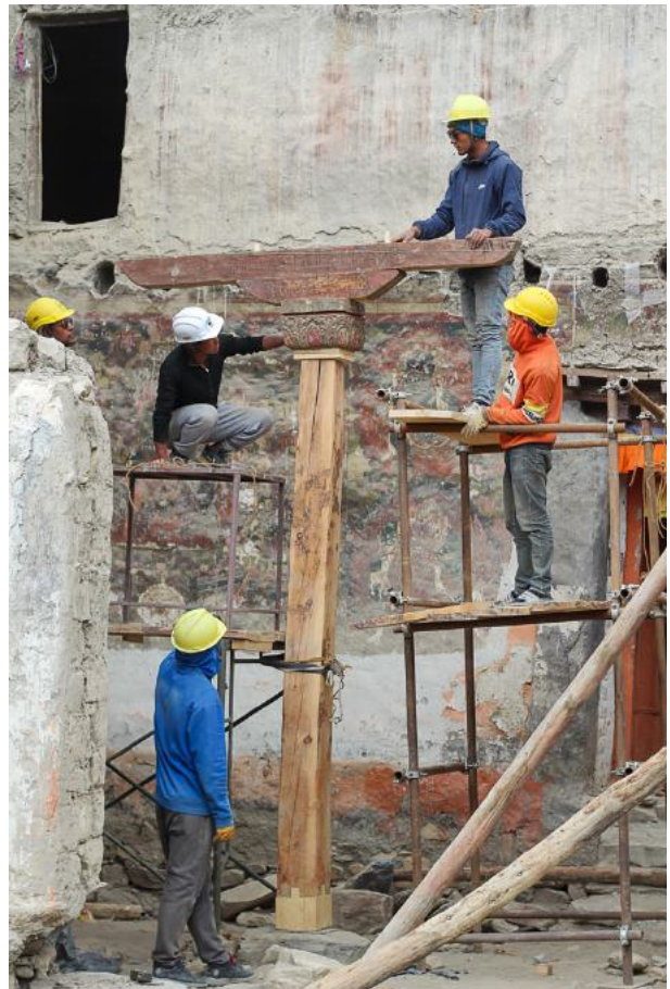
Figure 15: The old pillar with extension is placed on the new bedrock for reconstruction.
