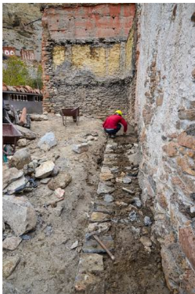
Figure 25: Constructing a stonewall along the building to consolidate its foundation.
