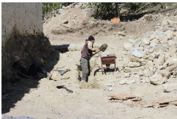
Figure 50: Digging a drainage at a distance to the temples walls.
