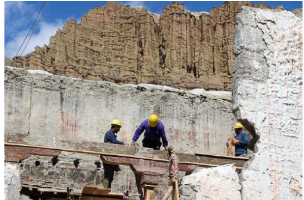
Figure 17: Here the laying of the beam is prepared by first placing the boards lying underneath it.
