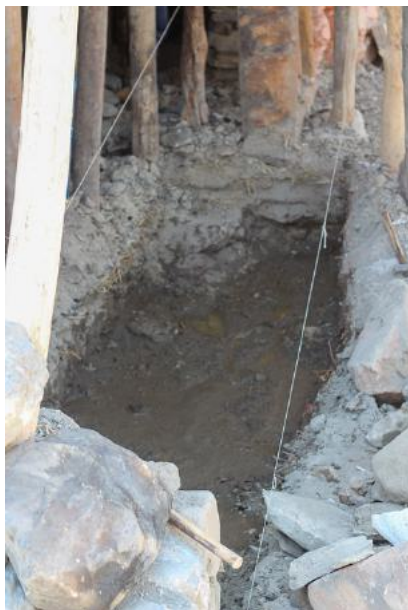
Figure 40: Preparing the foundation for the new corner wall.
