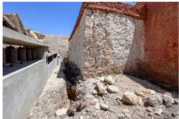
Figure 24: The most precarious parts of the foundation in the northwestern corner of the building.
