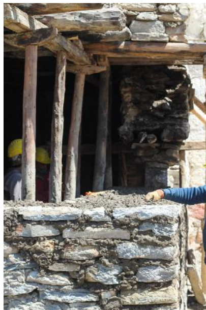
Figure 40: Preparing the foundation for the new corner wall.
