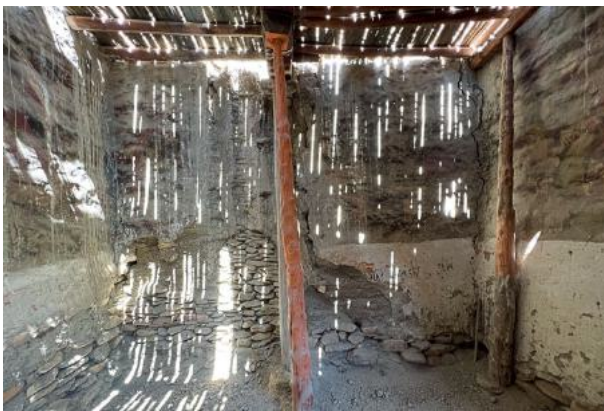
Figure 9: View of the entry hall wall with severely damaged murals during dismantling of the upper floor.
