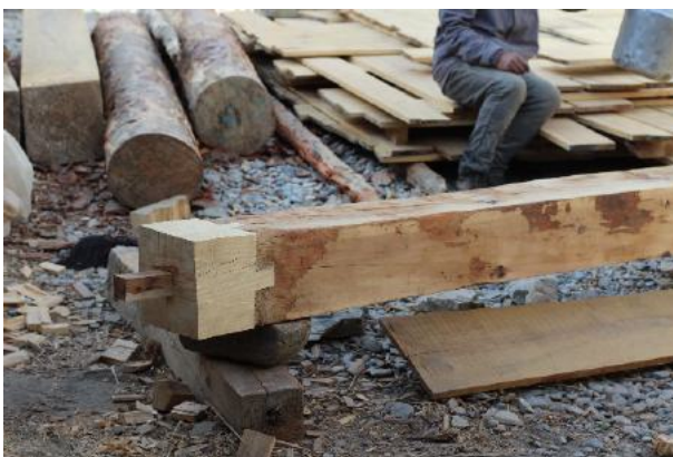
Figure 11: The original beam holding the porch was lengthened by adding a new bottom section.
