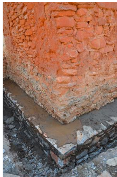
Figure 25: Constructing a stonewall along the building to consolidate its foundation.
