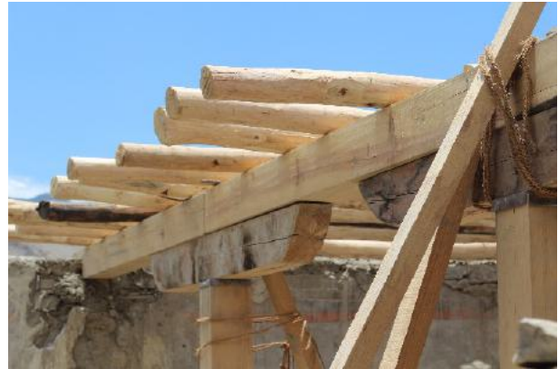
Figure 32: Assembling an old capital on top of a new beam on the top floor, note that their connection is reinforced.
