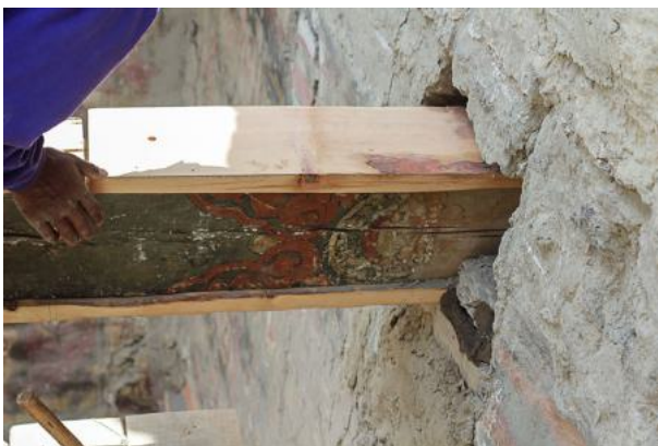
Figure 19: Placing the beam on the new support inside the wall.
