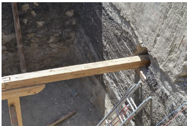
Figure 30: Placing the beam on new wall support.
