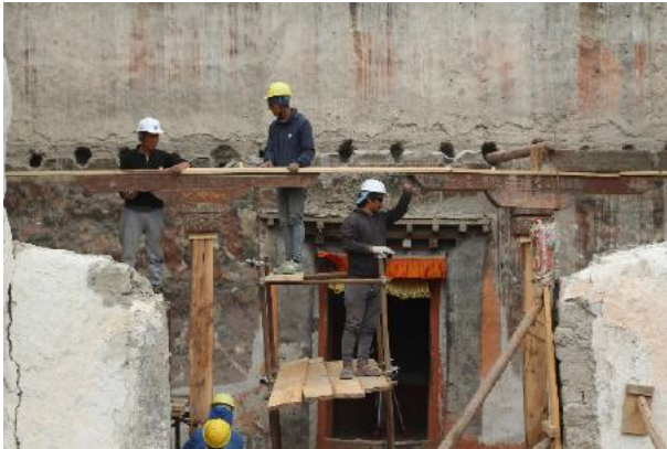
Figure 17: Here the laying of the beam is prepared by first placing the boards lying underneath it.
