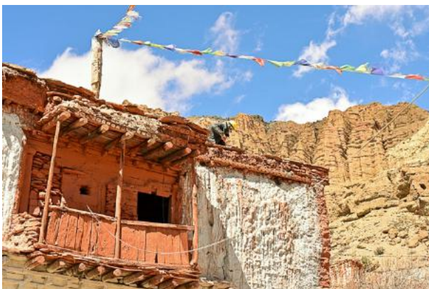
Figure 5: Dismantling of the porch area started from roof.
