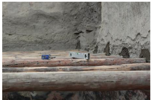
Figure 20: The joists are being refitted into the existing openings not to harm the wall paintings.
