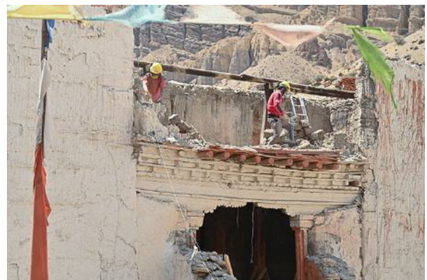
Figure 6: Then the entire often restored and poorly constructed balcony was dismantled.
