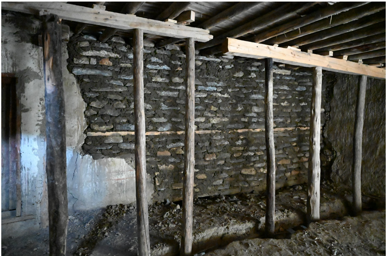
Figure 12: The second floor of the newly constructed wall from the interior.
