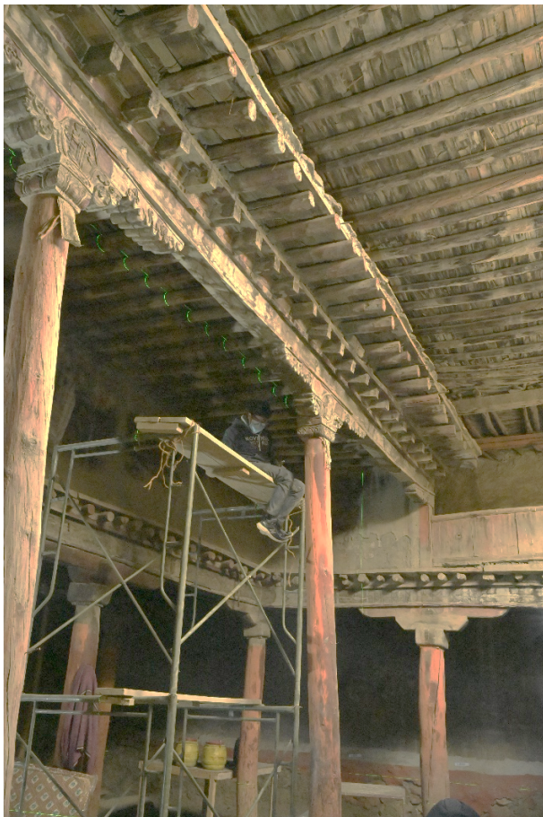
Figure 21: Taking detailed measurement of the capital on one of the long columns and discussing the measurements on site.
