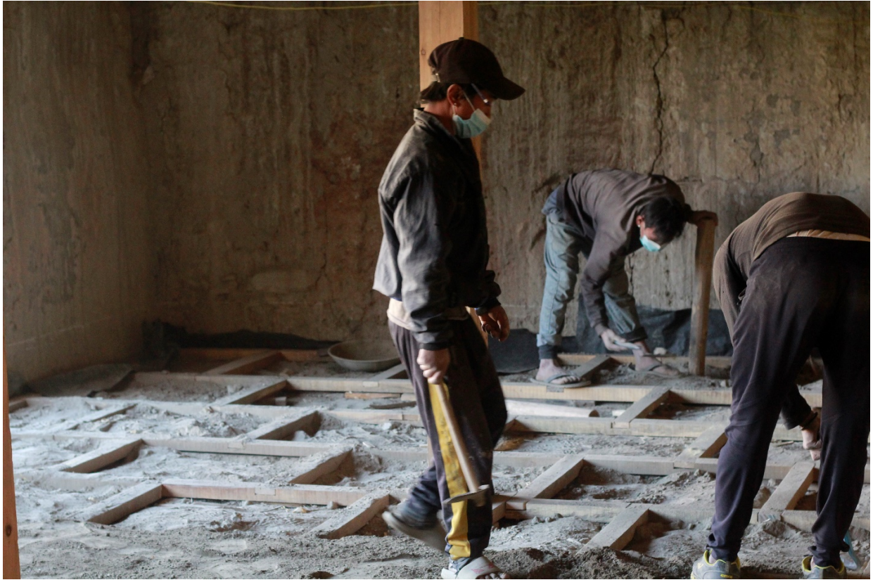
Figure 17: Laying out the wooden batten and mud for flooring.
