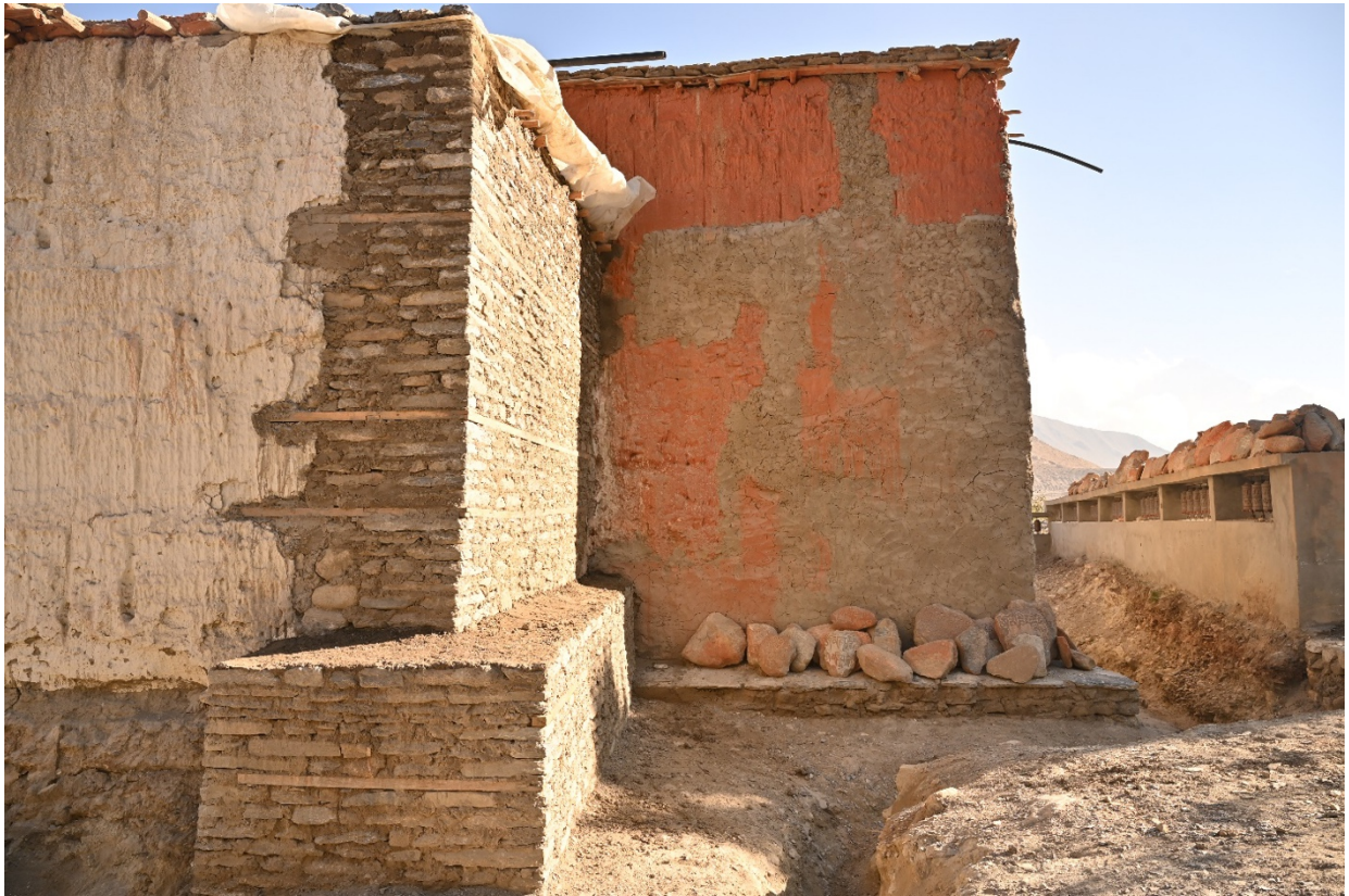
Figure 13: Northwest corner wall after completion.
