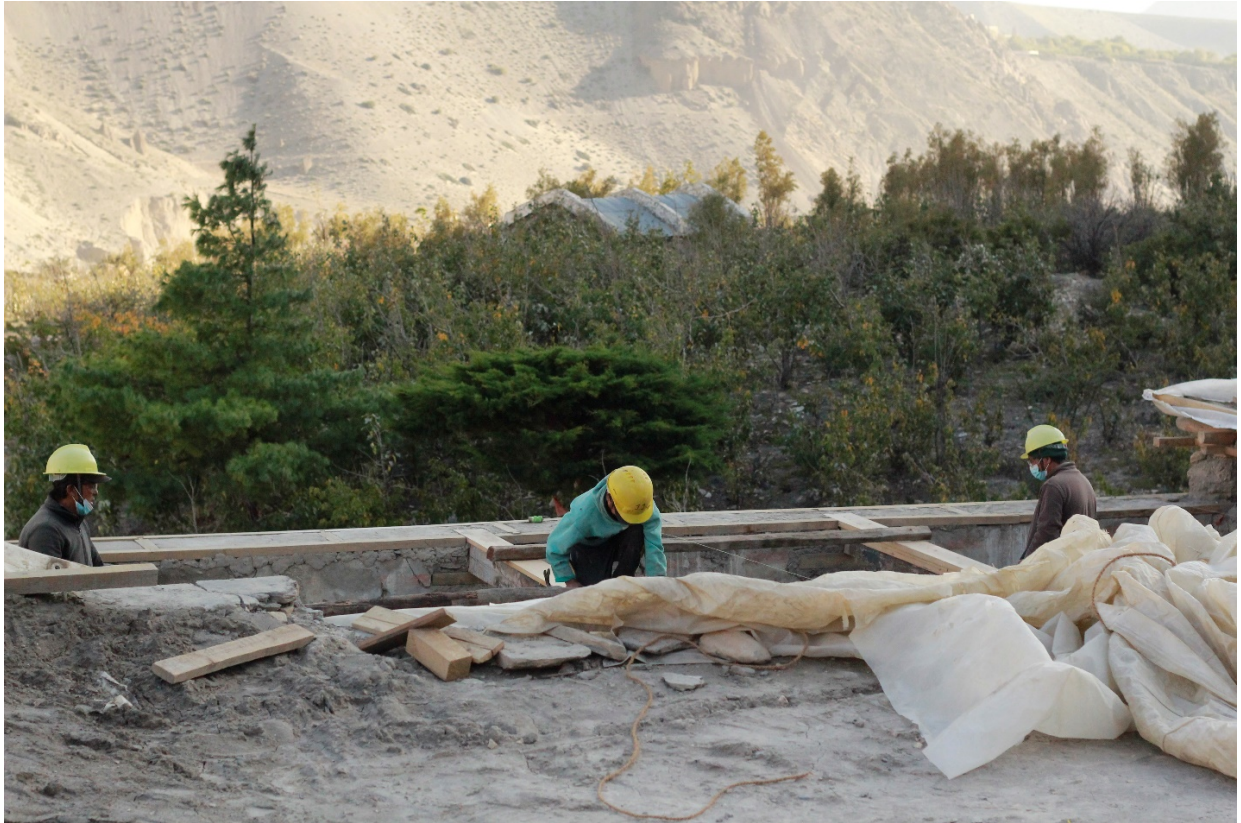
Figure 14: Installing the temporary roof above the south wing.
