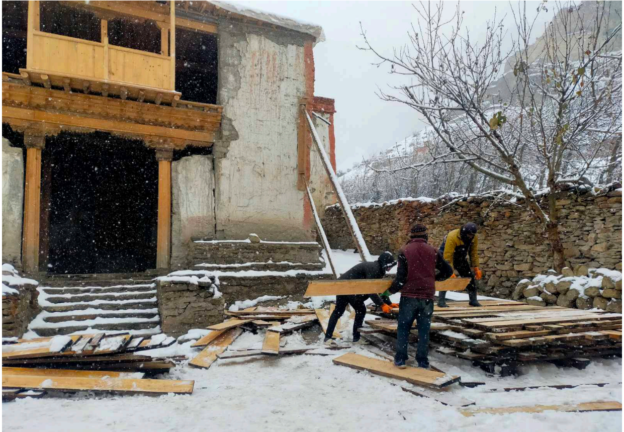
Figure 25: Stacking the wood properly.
