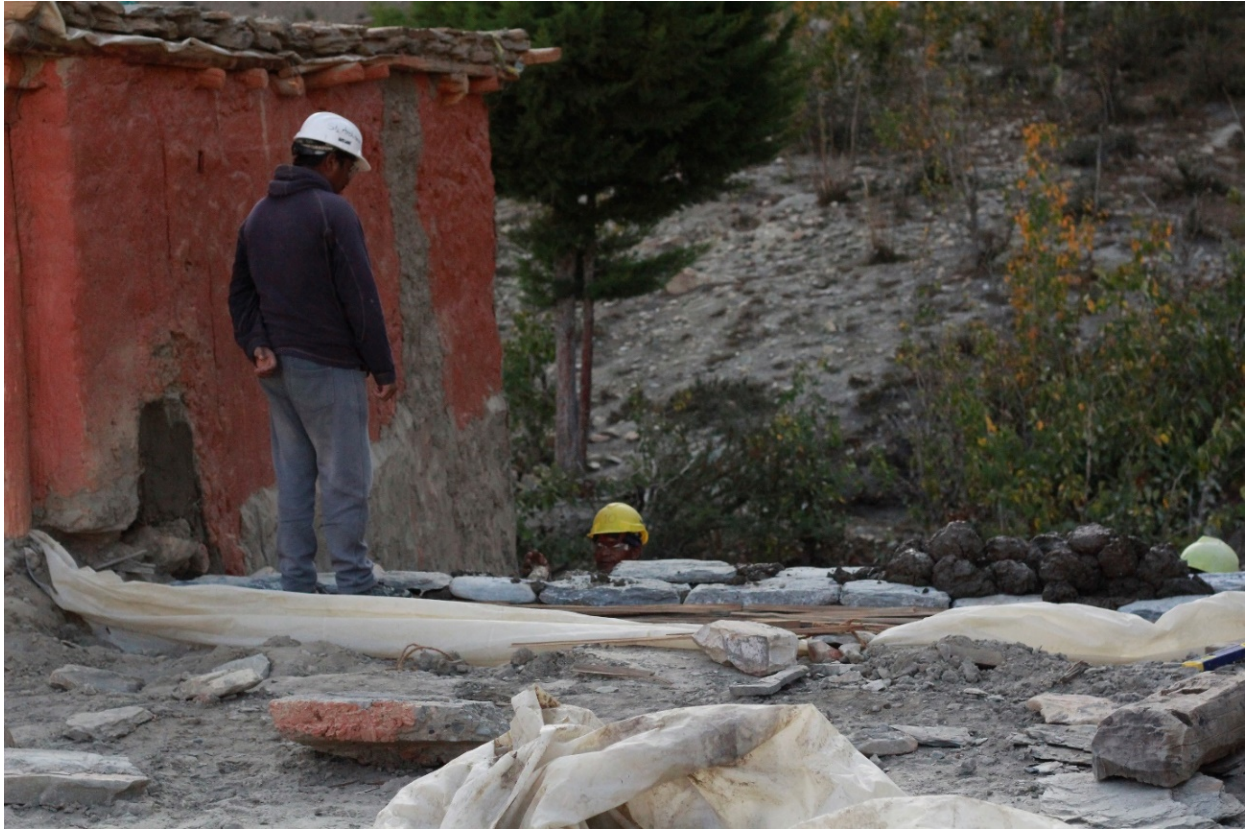
Figure 11: Installing the temporary roof above the new northwest corner wall.
