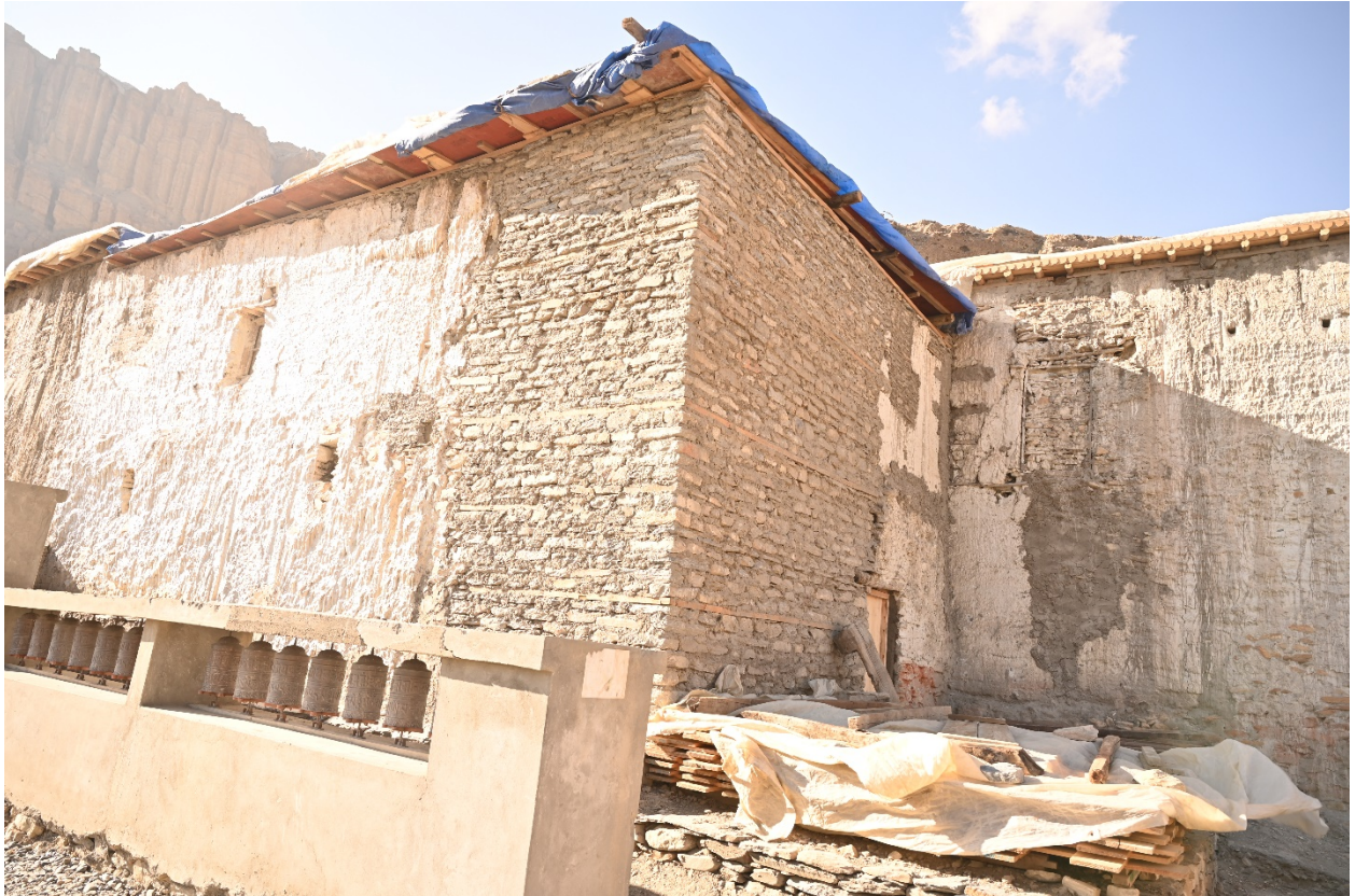
Figure 16: Temporary roof after completion.
