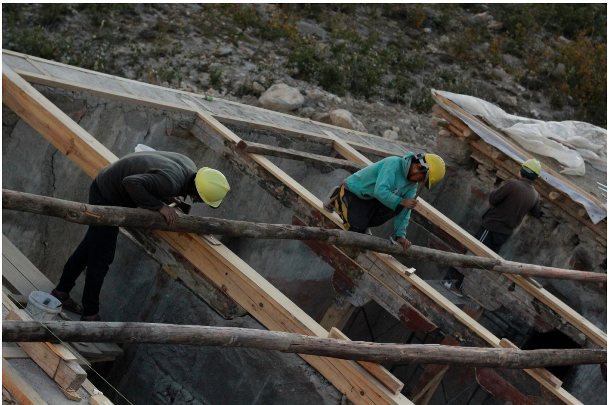
Figure 15: Installing temporary roof at south wing.
