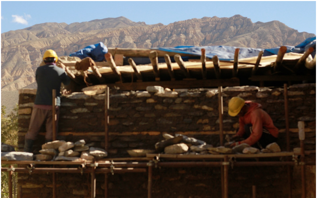
Figure 10: Reconstructing the northwest corner wall with wall ties.
